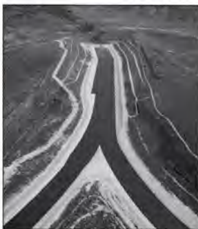
The Tehachapi Afterbay is where the West and East Branch bifurcate.
