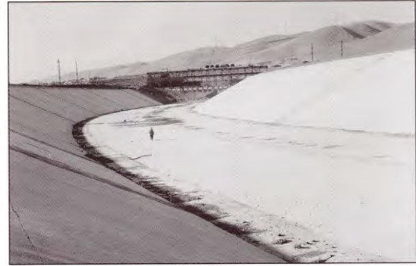
Construction was completed on the largest section of the Aqueduct in 1968. Part of the San Luis Canal, the section measures 200 feet wide with a water depth of 33 feet.
