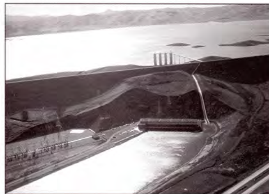
San Luis Dam impounds the largest off-stream storage reservoir in the United States – just over 2 million acre-feet.
