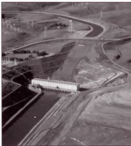
Located in the southern portion of the Sacramento-San Joaquin Delta, Banks Pumping Plant marks the beginning of the California Aqueduct.
