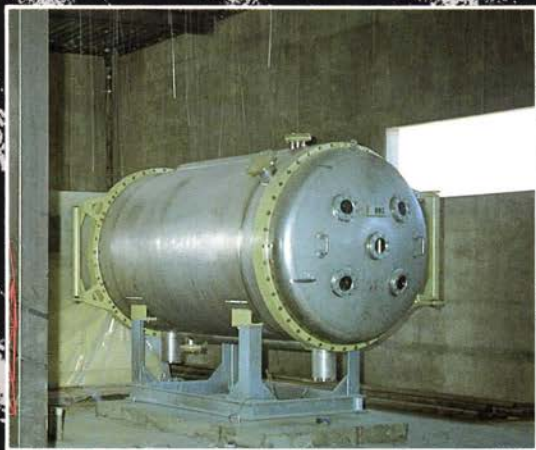
Generators produce ozone to disinfect water coming into the plant.
