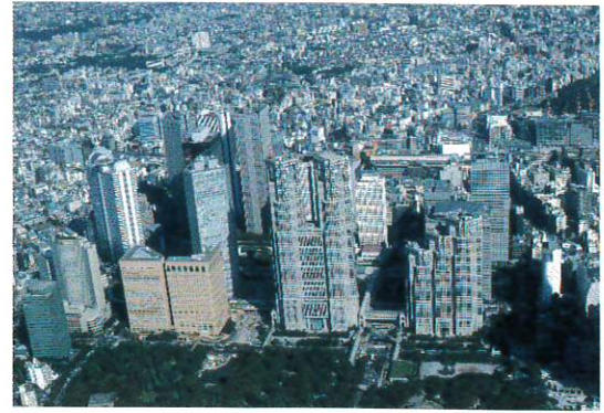
Shinjuku office buildings in Tokyo where reclaimed water is used for toilet flushing (Credit: Tokyo Metropolitan Government)
