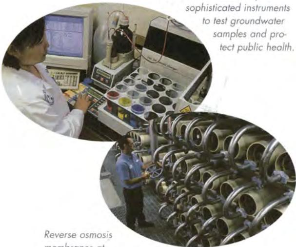
*Reverse osmosis membranes at OCWD's Water Factory 21 are the final purification step in turning wastewater into high-quality purified water—meeting drinking water requirements—that can be injected into the groundwater basin to prevent seawater contamination of Orange County's drinking water.*
