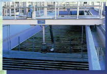
Carbon and sand filter beds
