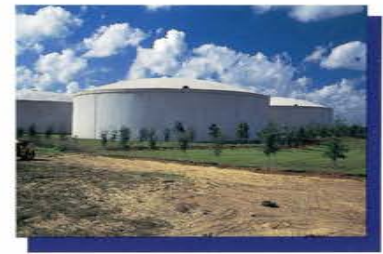
Distribution center ground storage tanks
