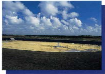
Rapid infiltration basin
