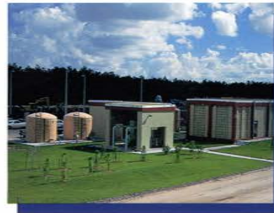
Chlorination facility for disinfection
