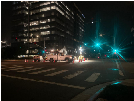
Workers complete utility work along Executive Drive for the Morena Northern Pipelines and Tunnels project (December 2021).
