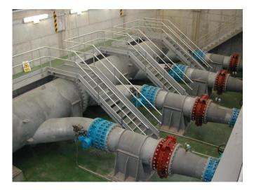
Figure 3. Reclaimed water pumping station for in-stream flow augmentation and agricultural irrigation.
