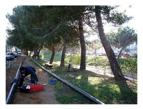
Figure 3. Construction of Tossa de Mar reclaimed water distribution network in 2007.
