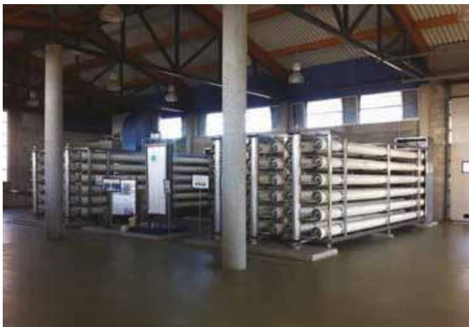
Reverse osmosis in the Torreele advanced water treatment plant, Belgium. Photo by Sandra Ryan
