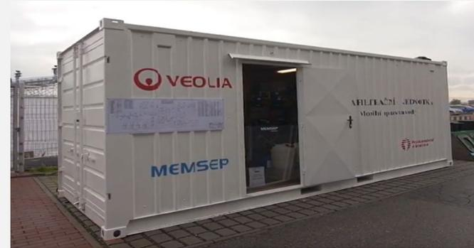
The treatment process comprises classical coagulation, followed by ultrafiltration and reverse osmosis, where ultra-fine synthetic membranes serve as a filter that lets water pass through and retains suspended solids and other substances such as micro-organisms and viruses.
